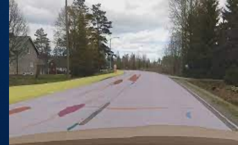
Road Condition Detection
